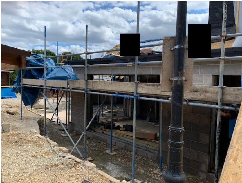
Roof and Ground Floor extension
