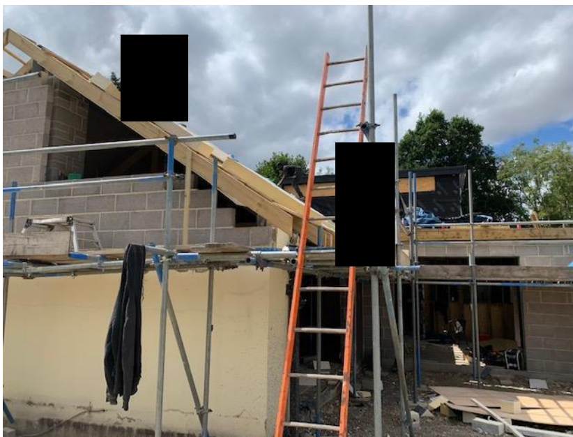
Rear elevation and Dormer
