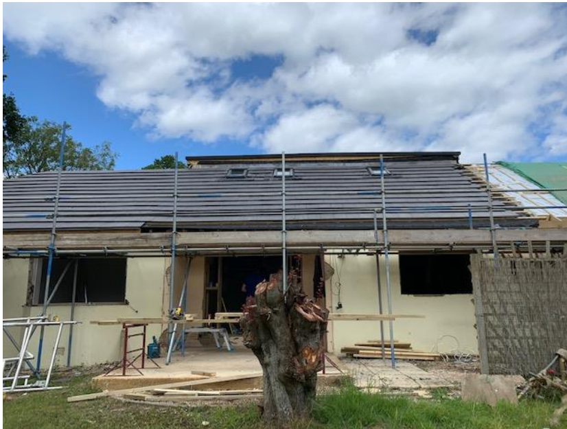
Front Elevation showing Dormer above roof ridge - 1
