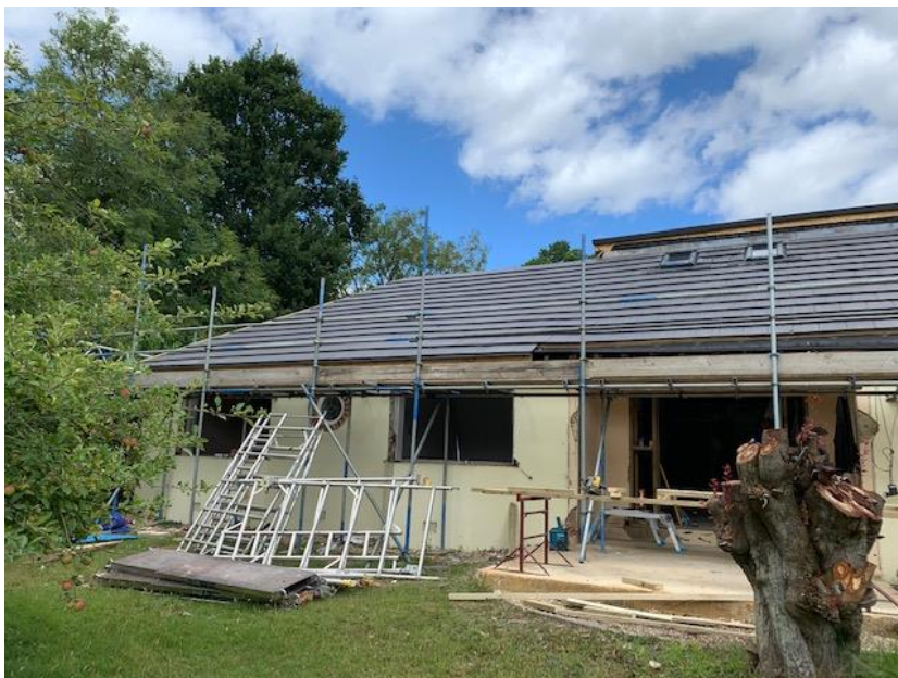
Front Elevation showing Dormer above roof ridge - 2
